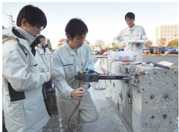
Inspection technology of bridge girder
